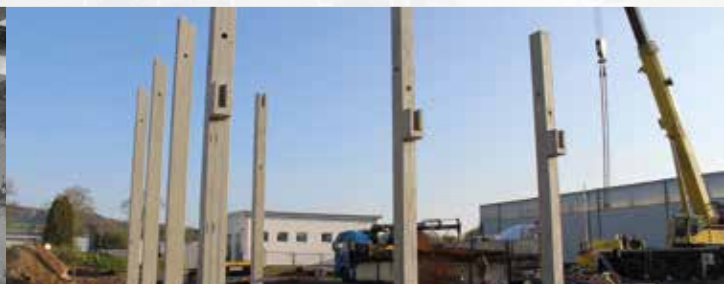
New Works III in Fröndenberg (as of April 2018)
